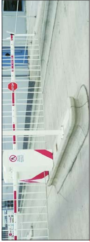
HIGH CONTAINMENT CURB 1500MM FROM EDGE
