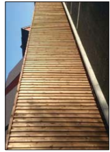
ERECTOR OF ACOUSTIC SCREENS
